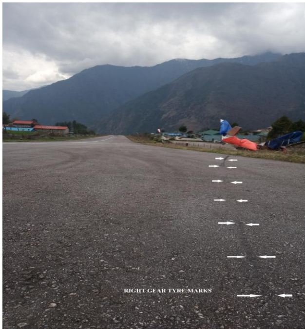
Figure 5 Tyre mark on the runway and aerodrome inner perimeter fence damage
